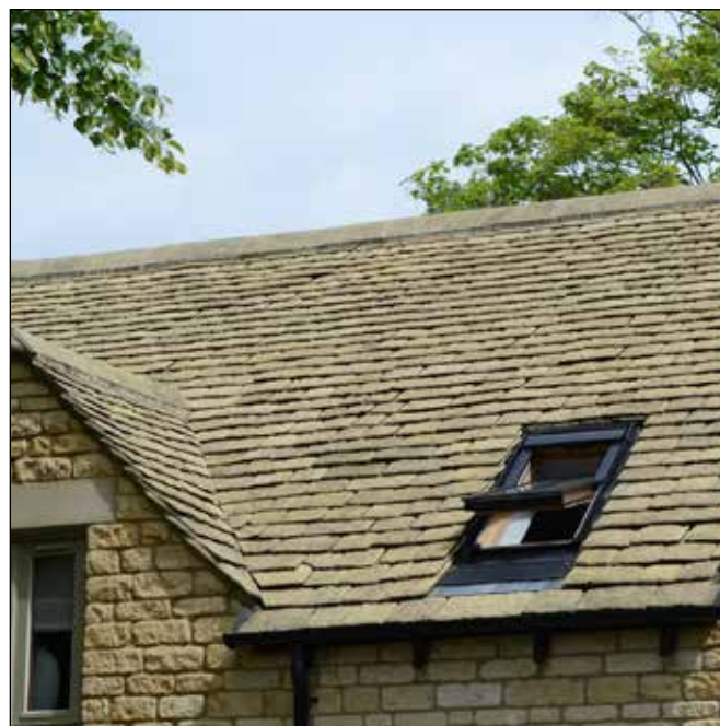
Fig. 7 Artificial stone slate roof with flush roof-light
