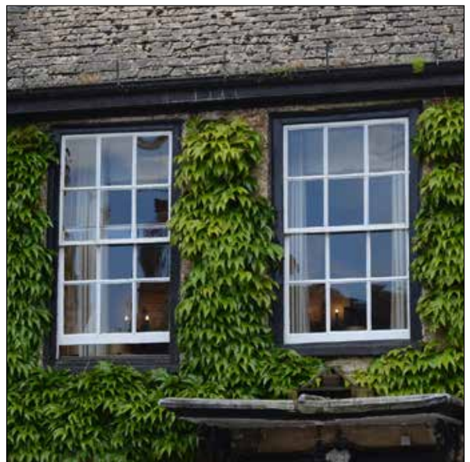
Fig. 2 Traditional vertical sliding sash windows
