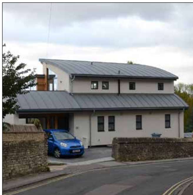
Fig. 5 Standing seam roof on recent house in Woodstock
