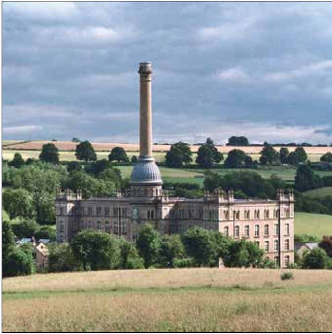
Fig. 5 Chipping Norton CA - key view of Bliss Mill
