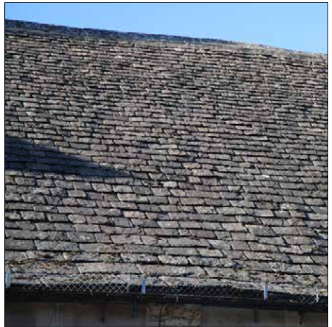
Fig. 2 Natural stone slates laid in diminishing courses
