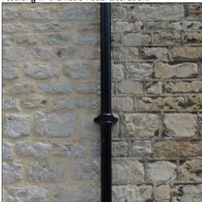
Fig. 8 Stonework should always be repaired with care
