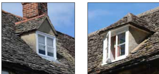
Fig. 4 Traditional local gabled and hipped dormers
