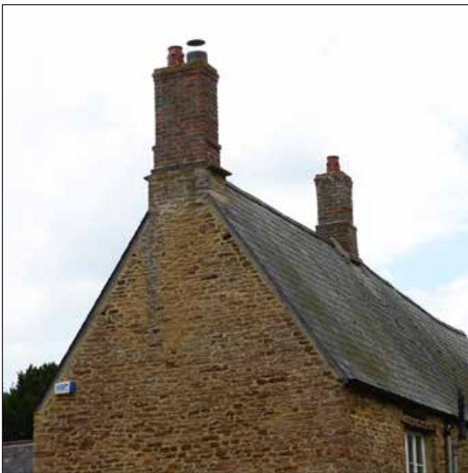
Fig. 1 Locally characteristic steeply pitched roof
