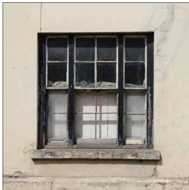
Fig. 7 Original windows should be retained and repaired
