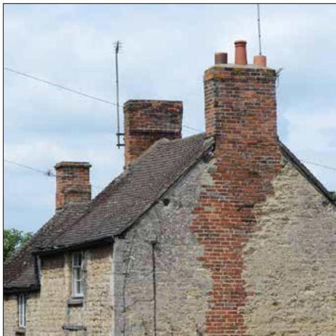
Fig. 8 Traditional brick chimneys in Woodstock
