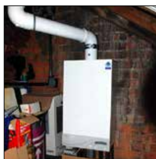
Fig. 11 Combi-condenser boiler, and flue next to chimney
