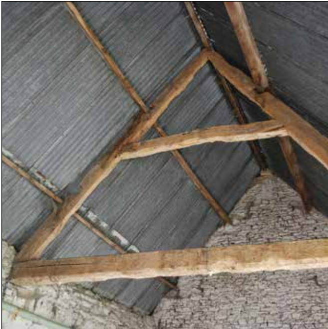
Fig. 7 Original roof trusses should be retained
