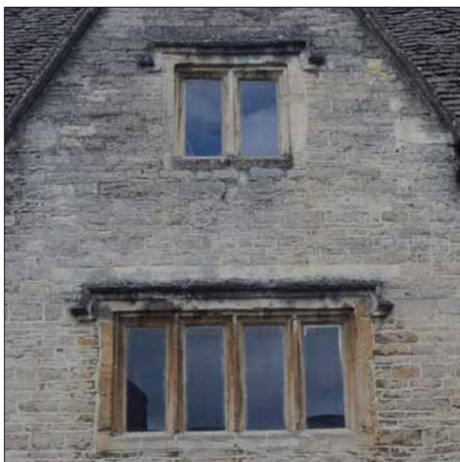
Fig. 3 Traditional C17 stone mullion windows
