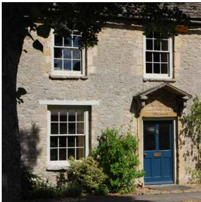
Fig. 2 Listed house in Witney
