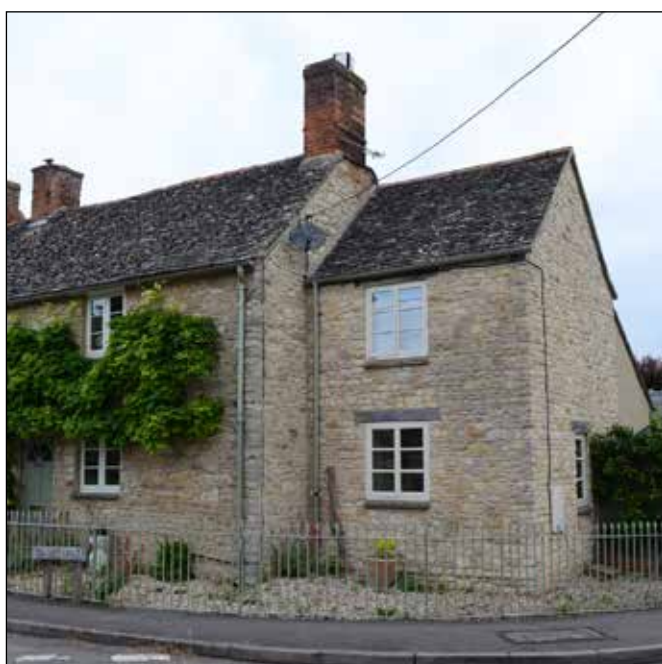
Fig. 1 Two-storey side extension to a traditional house
