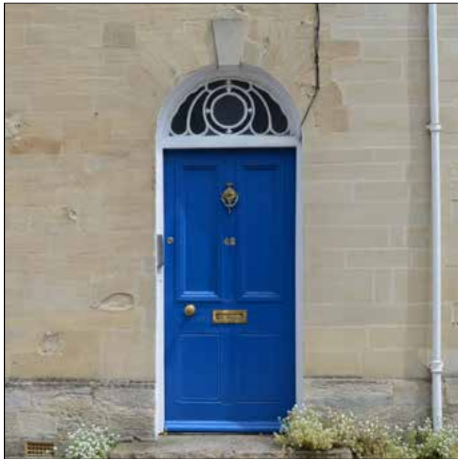
Fig. 9 A traditional paneled entrance door
